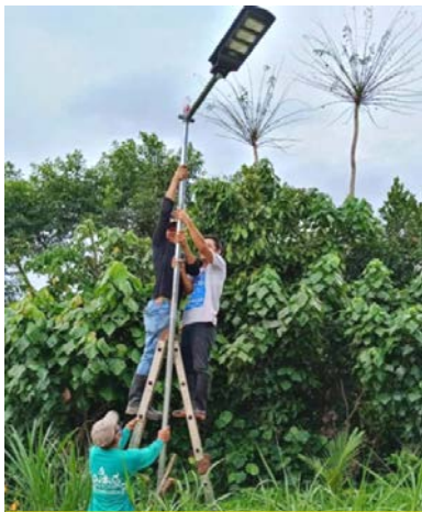
Installation of Additional Solar Street Lights
