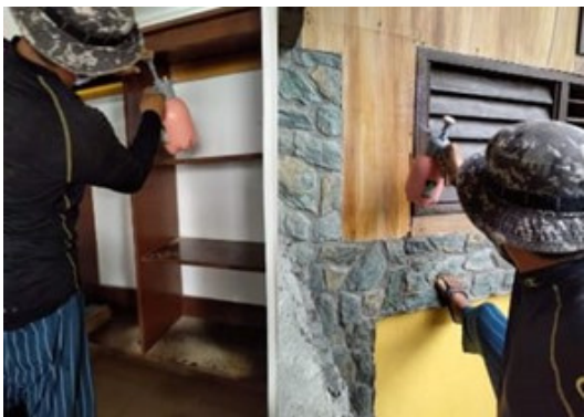
Sprayed poison for termites
