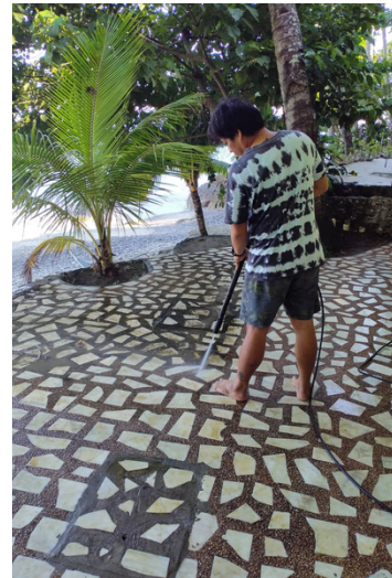
Removed algae using high pressure
