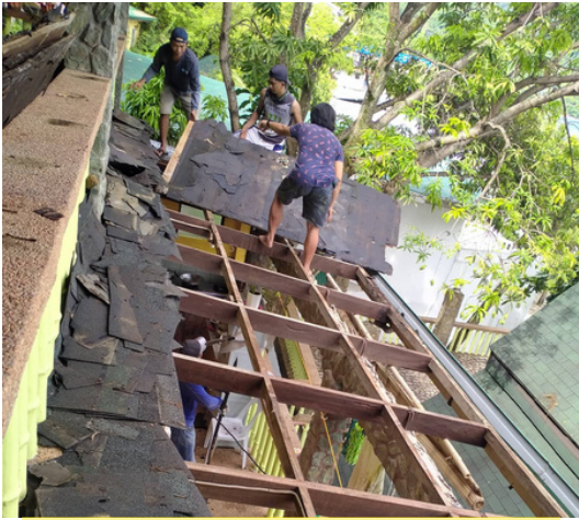
Repaired and replaced damaged roofs
