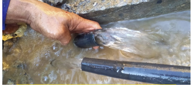
Pipe from the pump had been repaired
