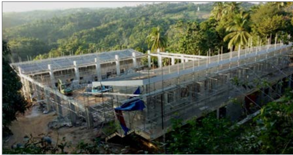
Multi Purpose Building Construction (MPB)
